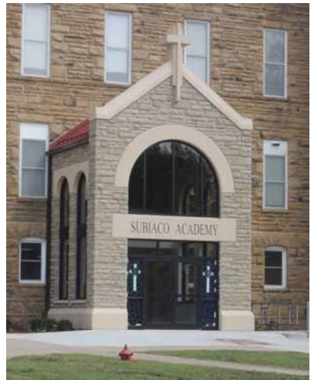
A new front entrance to the Academy was part of the campaign
